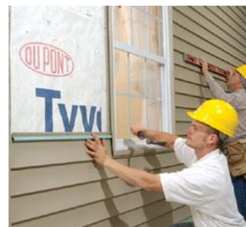
DuPont’s Tyvek house wrap under typical vinyl siding.
